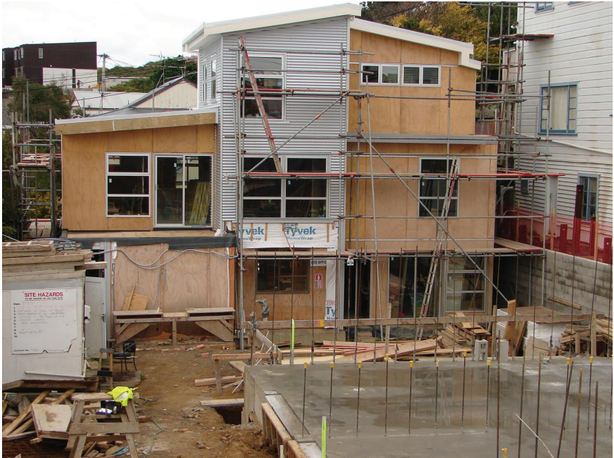
Construction of Stoke Street project
