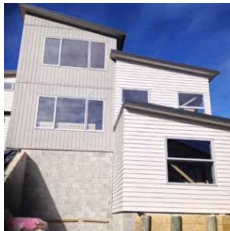
Vennell Street nearing completion
