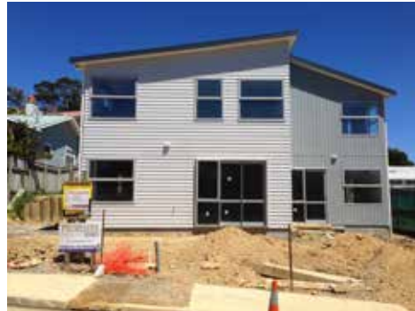
Vennell Street near completion
